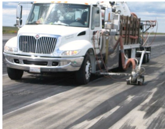
Rubber removal using ultra-high waterblasting with vacuum recovery
