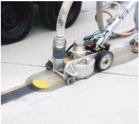
Lines Stripe Removal using ultra-high waterblasting – approved for lead paint removal
