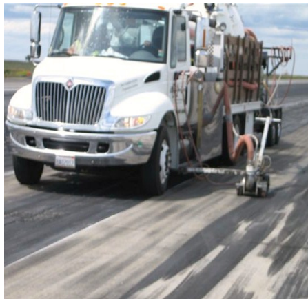
Rubber removal using ultra-high waterblasting with vacuum recovery
